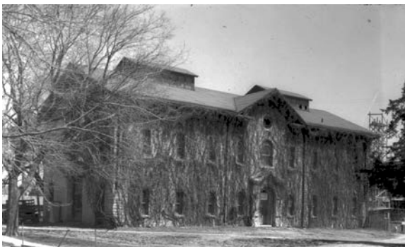
Figure 1. Farm Machinery Hall - ca. 1948.
